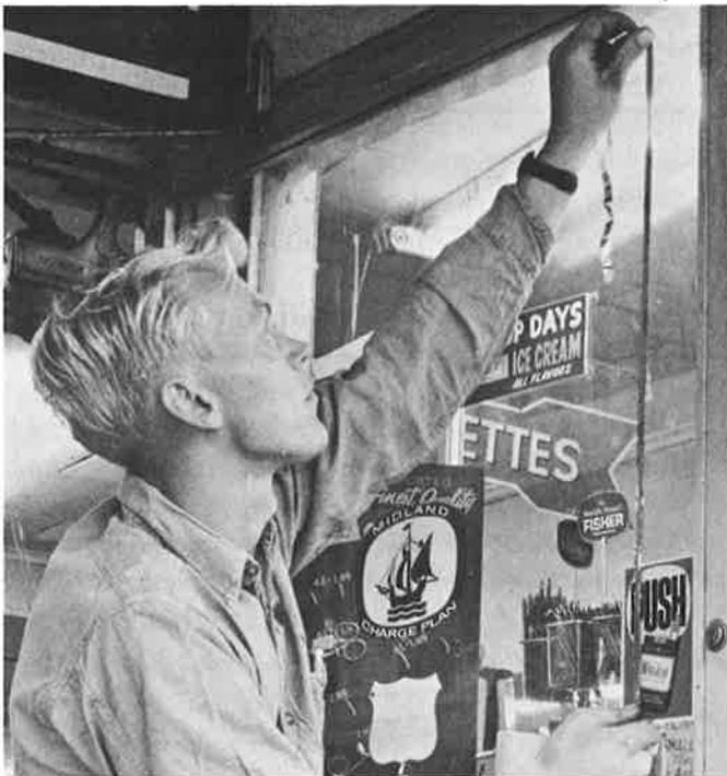
This tape being installed as part of a burglar alarm system in drug store, by a Doyle mechanic, becomes part of the dual circuit which effectively deters and stops burglaries.
